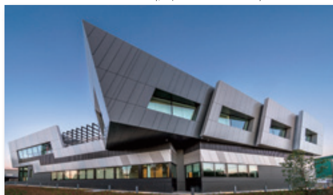
Exterior, Equinix SY4 Sydney IBX® Data Center
