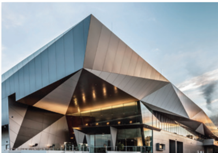
Exterior, Equinix ME1 Melbourne IBX® Data Center
